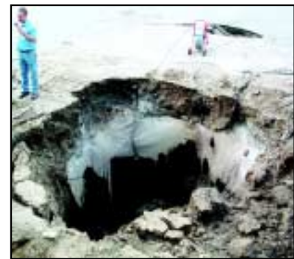
Figure 5-7. Ice-rich permafrost thawing and surface and groundwater intensive flow created this thermokarst pit in a parking lot in Fairbanks, Alaska (photo by V. Romanovsky).
